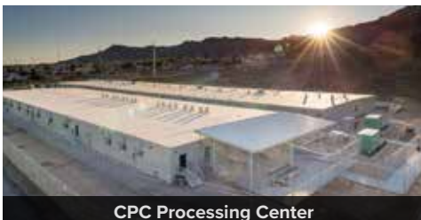
CPC Processing Center
