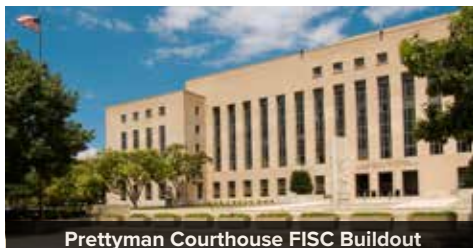
Prettyman Courthouse FISC Buildout
